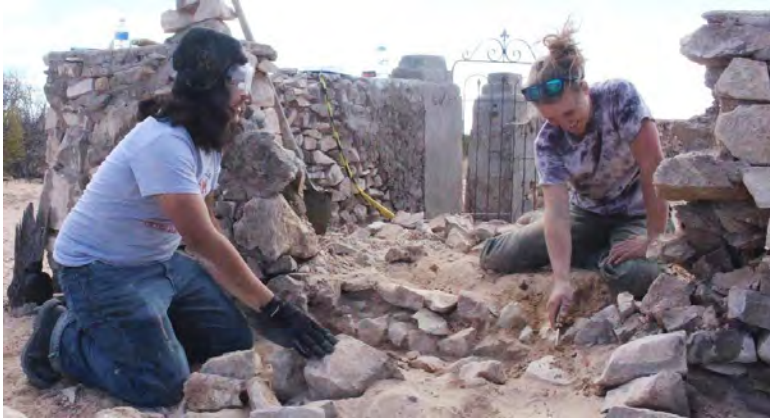
Crew working on repair of perimeter wall
